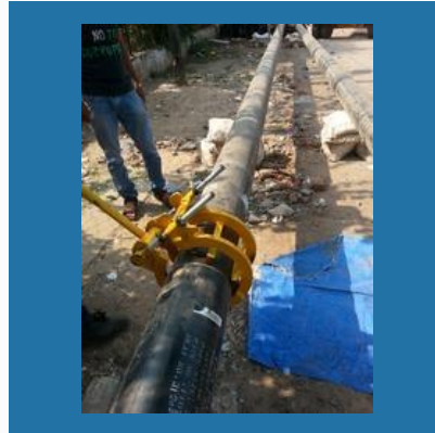
External Pipe Line Up Clamp
